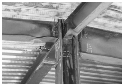
(b) Symmetrical (non-sway) mode of buckling
